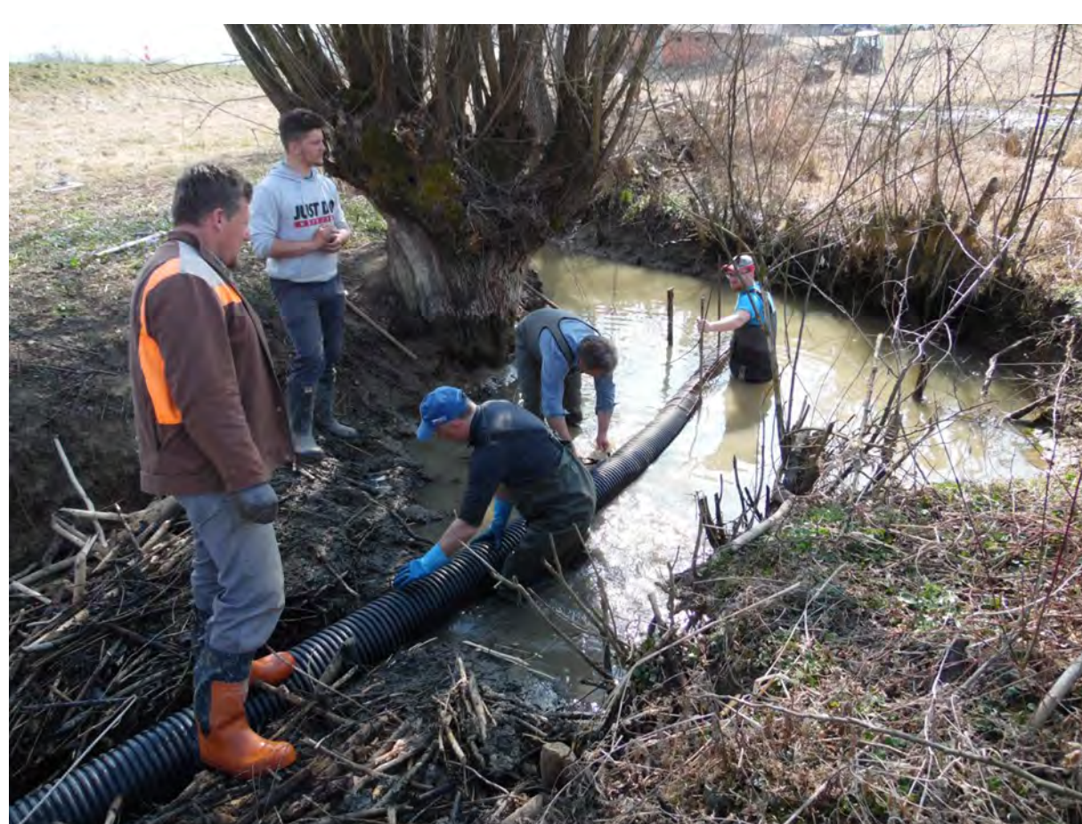
Beaver deceiver “BOBROBRAN” installation on a smaller stream.
